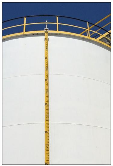
tank is full, the float reaches the upper part of the tank while the index points to the lowest position of the graduated scale. The few moving parts and the very low speed make this level indicator a reliable instrument that is no subject to failure. Moreover, the simplicity of the measuring system makes monitoring and maintenance possible even for nonspecialists.
